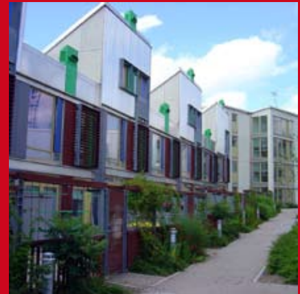
High density Townhouse: In Amsterdam (left) and the Greenwich Millennium Community in London.
